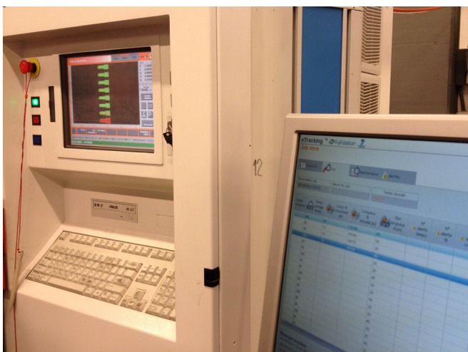
Figure 2: An Electric Discharge Machining (EDM) device at GF Agie-Charmilles
